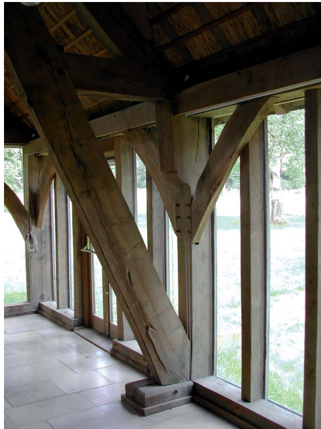
Fig. 4.8 Traditional oak construction – Great Oak Hall, Westonbirt Arboretum, Gloucestershire. Architects: Roderick James Architects. Photograph: Arthur Lyons
