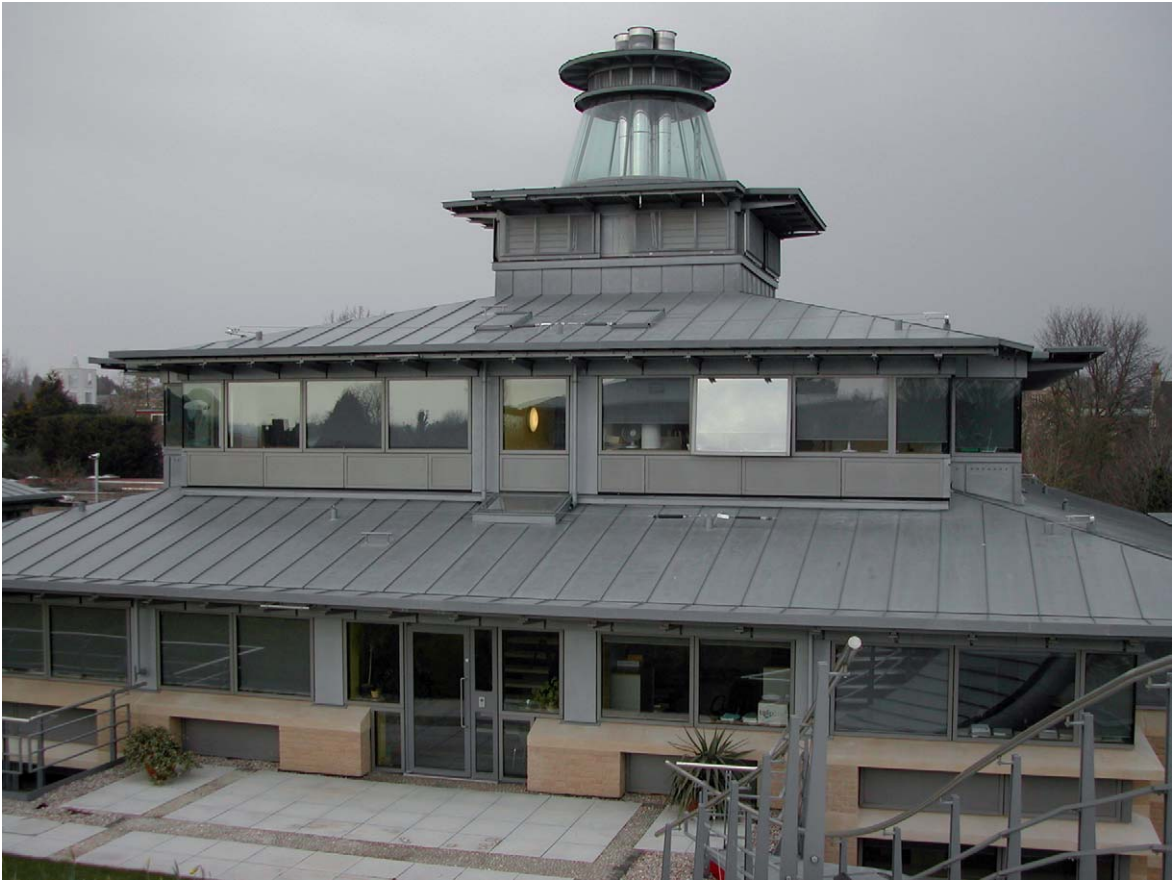
Fig. 5.28 Zinc alloy roofing – Centre for Mathematical Sciences, University of Cambridge. Architects: Edward Cullinan Architects. Photograph: Arthur Lyons
