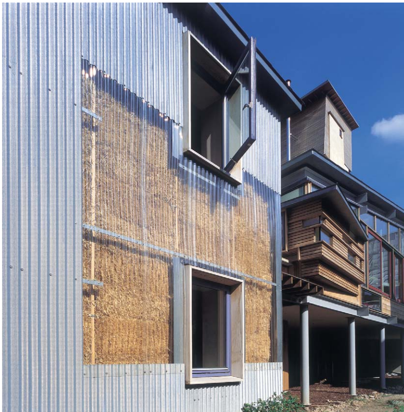
Fig. 15.2 Straw bales in construction. Architects and Photograph: Sarah Wigglesworth Architects
