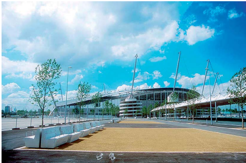
Fig. 5.3 Structural steelwork – Manchester City Stadium. Architects: Arup Associates. Photograph: Courtesy of Arup Associates
