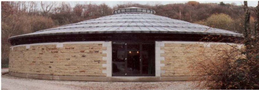
Fig. 9.10 Load-bearing stone masonry – David Mellor Cutlery Factory, Hathersage, Derbyshire. Architects: Hopkins Architects. Photographs: Arthur Lyons
