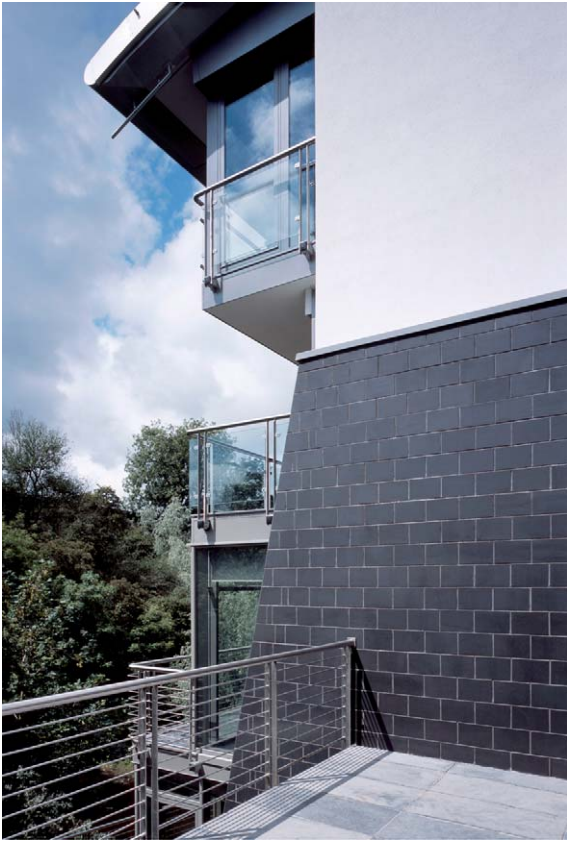
Fig. 2.9 Fairfaced blockwork – IDP Offices, Glasgow. Architect: IDP. Photograph: Courtesy of Ibstock Brick Ltd
