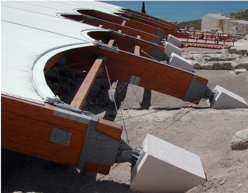
Fig. 4.22 Glued laminated-timber beams. Photograph: Arthur Lyons
