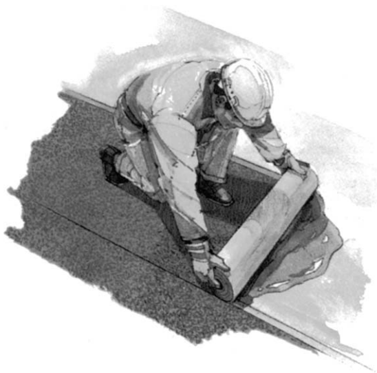
Torching-on high-performance roofing sheet
