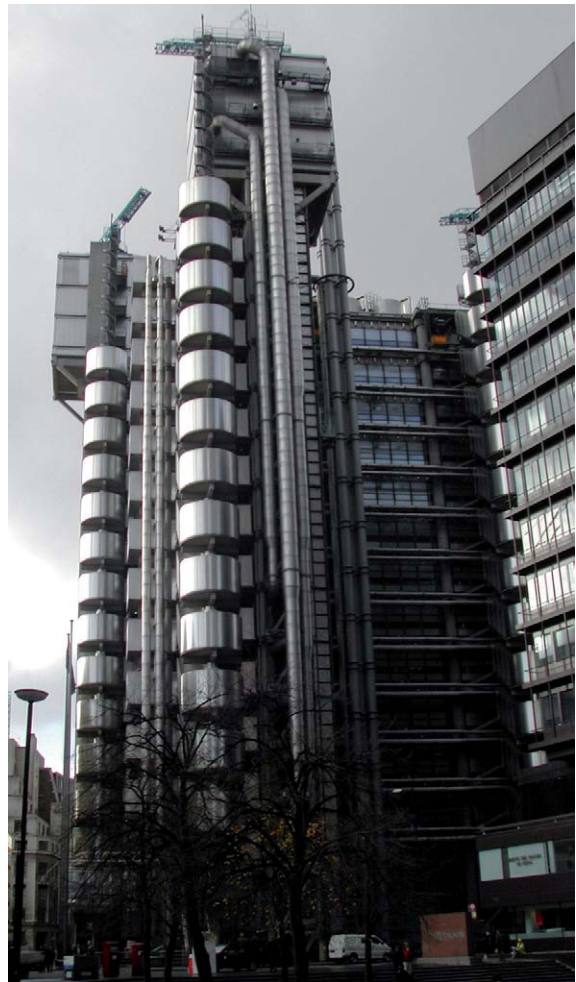
Fig. 5.16 Stainless steel construction – Lloyd's Building, London. Architects: Richard Rogers. Photograph: Arthur Lyons
