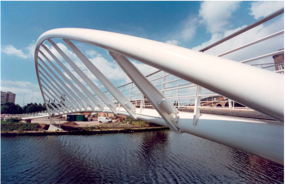
Fig. 5.10 Curved steel sections – Merchants Bridge, Manchester. Photograph: Courtesy of The Angle Ring Company Ltd
