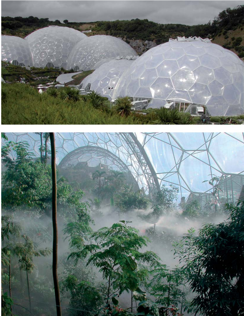
Fig. 10.14 ETFE – Eden Project, Cornwall. Architects: Nicholas Grimshaw and Partners. Photographs: Arthur Lyons and courtesy of Perry Hooper (interior)
