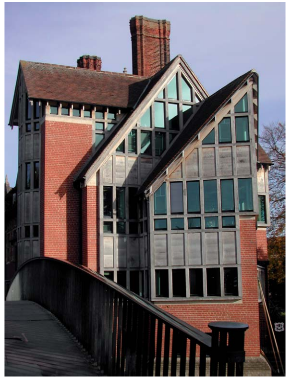
Fig. 4.7 Limed Oak – Jerwood Library, Trinity Hall, Cambridge. Architects: Freeland Rees Roberts. Photograph: Arthur Lyons
