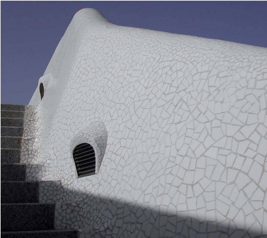
Fig. 8.11 Concert Hall, Tenerife and ceramic mosaic detail. Architect: Santiago Calatrava. Photographs: Arthur Lyons
