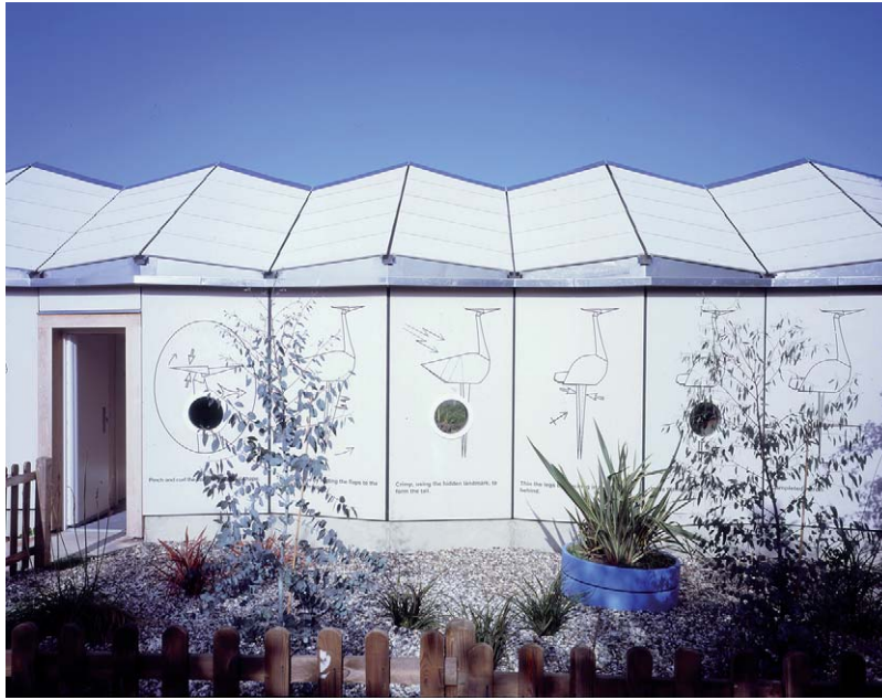
Fig. 15.3 Cardboard Classroom – Westborough School, Essex. Engineers: Buro Happold. Architects: Cottrell and Vermeulen. Photograph: Copyright Adam Wilson/Buro Happold
