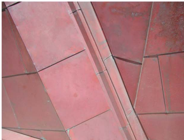
Fig. 5.20 Copper cladding – Swan Bells Tower, Perth Australia. Architects: Hames–Sharley Architects. Photographs: Arthur Lyons
