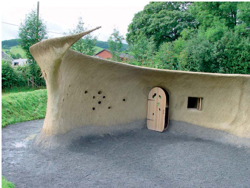
Fig. 15.4 Mud and straw construction – The House for Stories, Bleddfa Centre for the Arts, Powys, Wales. Architect: Tono Mirai. Photograph: Courtesy of Richard Weston
