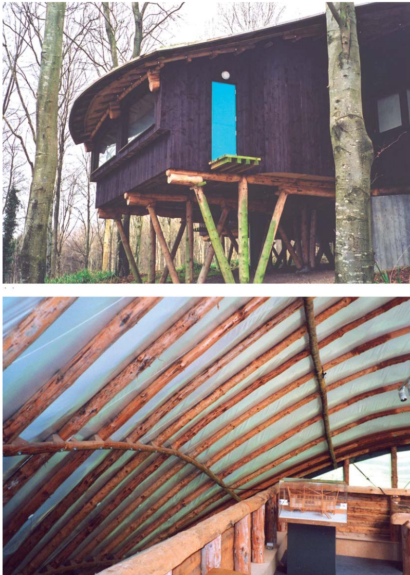
Fig. 4.16 Timber pole construction – Hooke Park, Dorset. Lodge (Edward Cullinan Architects and Buro Happold), and workshop interior (Frei Otto, Ahrends Burton & Koralek and Buro Happold). Photographs: Courtesy of Allan Glennie
