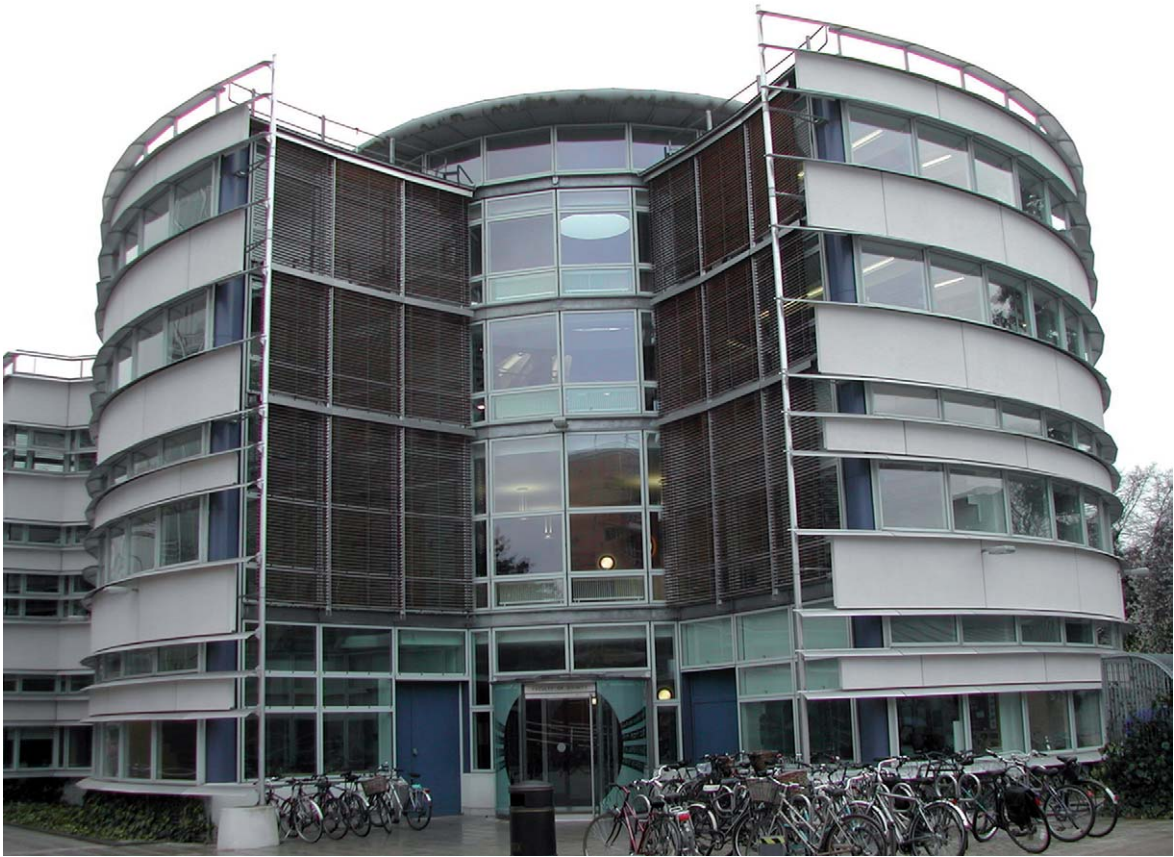
Fig. 5.17 Aluminium shading devices – Faculty of Divinity, University of Cambridge. Architects: Edward Cullinan Architects. Photograph: Arthur Lyons
